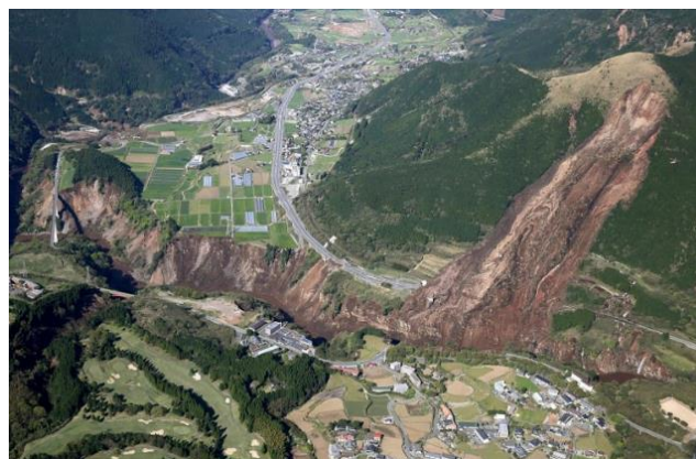
Figure 1.12 A landslide triggered by the Kumamoto earthquake, Japan 2016 ( https://blogs.agu.org/landslideblog/2016/04/18/kumamoto-earthquake-1/ )
