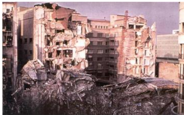
Figure 1.10 Partial collapse of a structure in Bucharest, Vrancea earthquake of March 4, 1977 ( https://www.igsu.ro/ )
